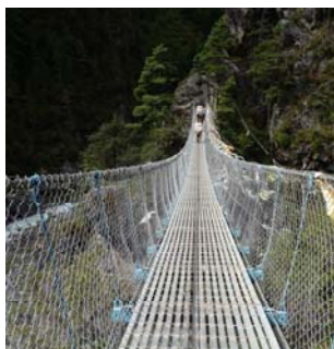
In suspense: trail bridge.
